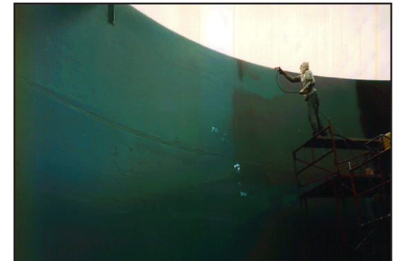
ARC S2 spray applied with airless system
