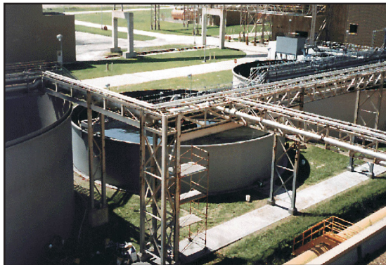
One of four tanks to be lined
